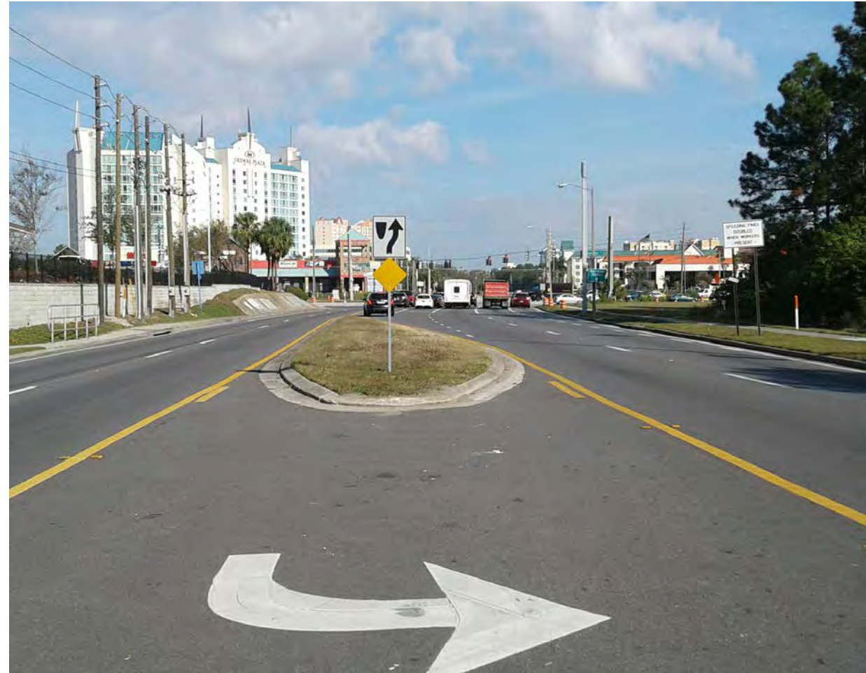
Universal Boulevard south of Sand Lake Road
