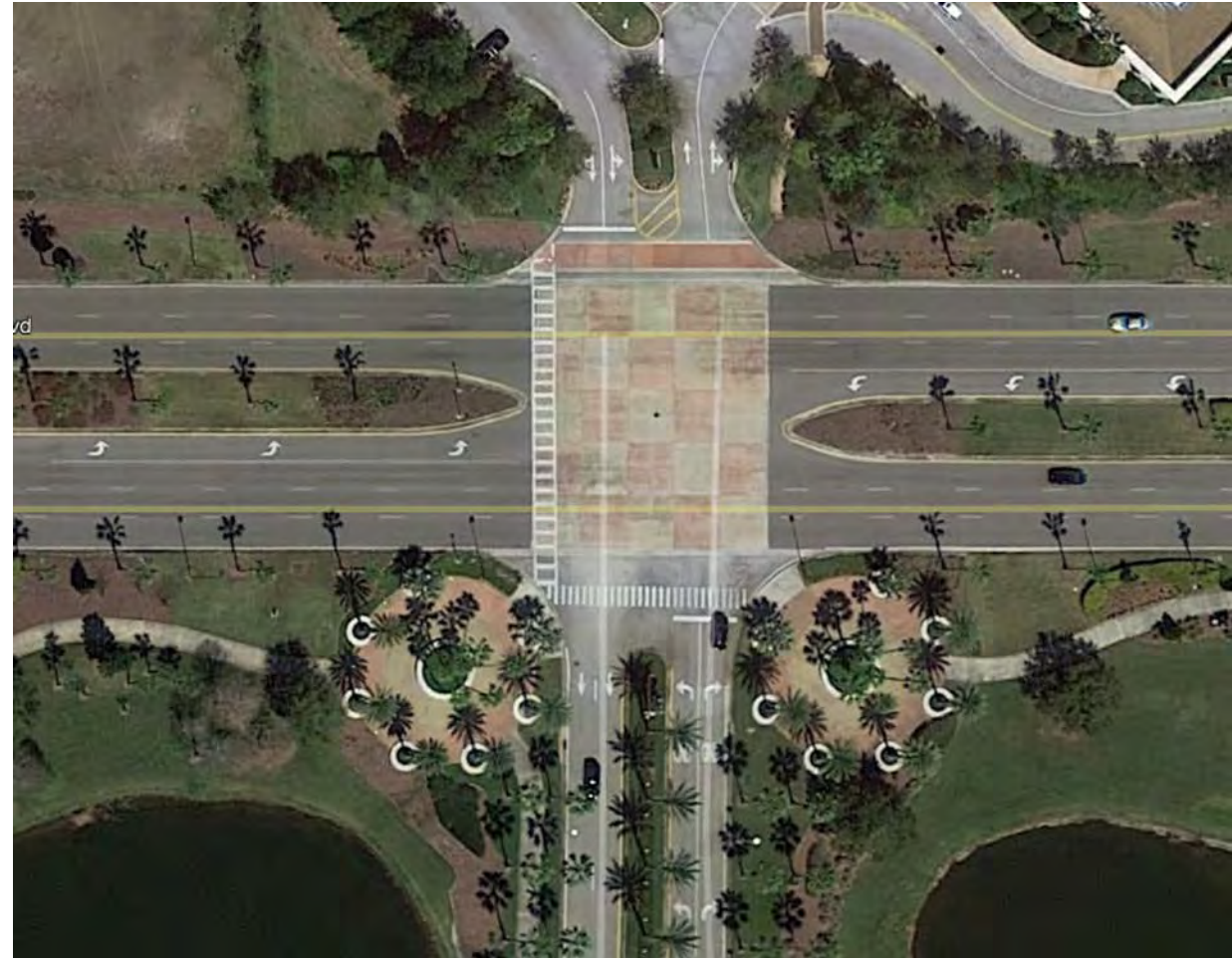
Universal Boulevard at OCCC North Concourse/Hilton Driveway
